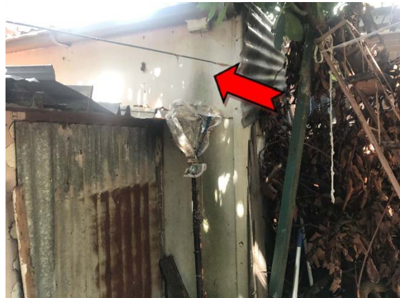
Photo 4. Exterior, store 2, wall cladding – asbestos-containing fibre cement sheeting.
