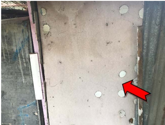
Photo 3. Exterior, store 1, wall cladding – asbestos-containing fibre cement sheeting.
