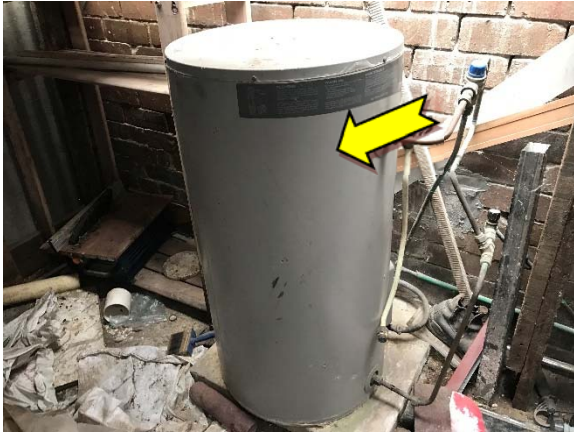
Photo 7. Exterior, eastern elevation, hot water heater – suspected SMF internal insulation.
